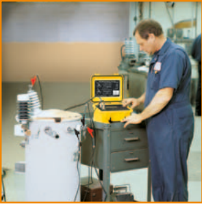
Measurement on a transformer in the workshop
